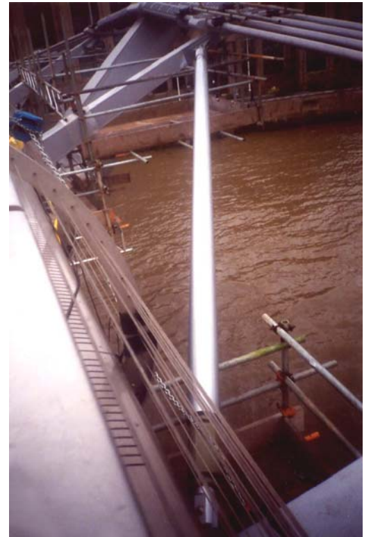
FIGURE 8 PIER DAMPERS
