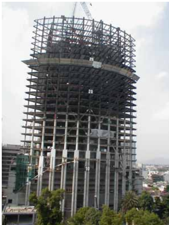
FIGURE 8 TORRE MAYOR BUILDING FRAME
