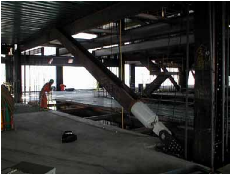
FIGURE 13 DAMPER INSTALLATION
