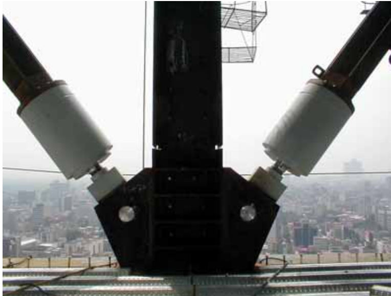
FIGURE 11 DAMPER INSTALLATION
