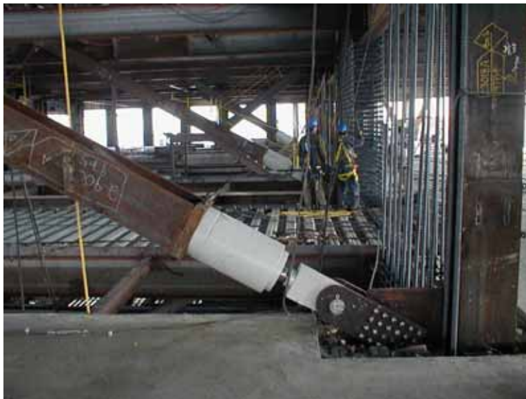
FIGURE 12 DAMPER INSTALLATION
