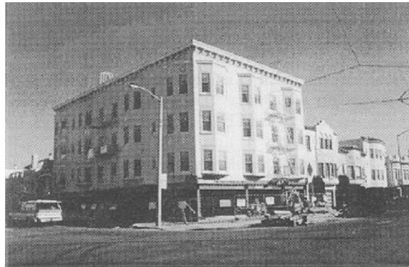
Figure 7. Photograph of four-story wood-framed apartment building seismically retrofitted with a sliding isolation system. (From Zayas and Low 1997, © Forest Products Society. Reproduced with permission.)
