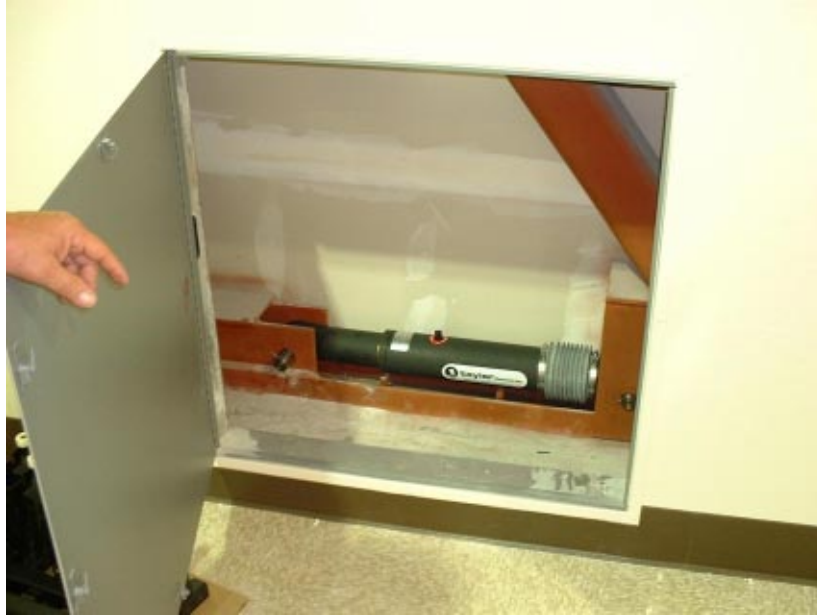
Figure 9. Typical damper installation.
