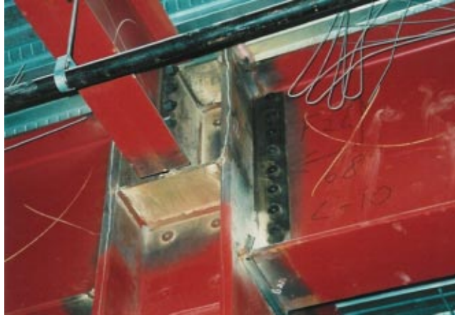
Figure 1. Typical existing moment-frame connection.
