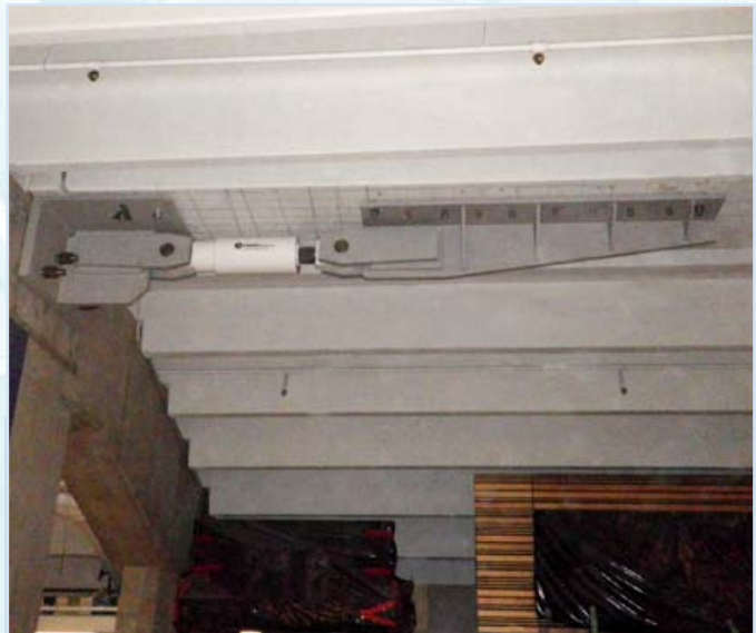
A finished damper installation by construction workers at site
