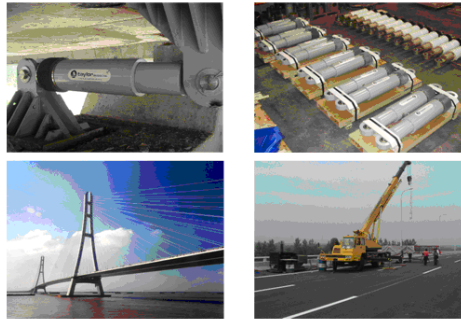
Fig. 1 Nanjing Yangtze river 3 rd bridge and 54 dampers
