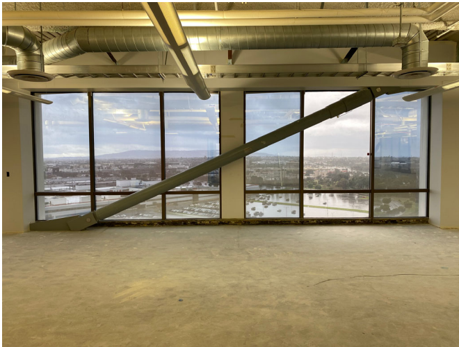
Photo 2. FVD in Longitudinal Direction of Building
