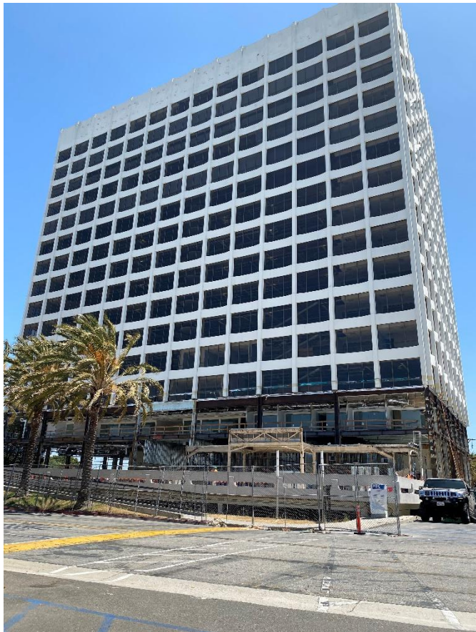
Photo 1. Exterior View of Building During Construction
