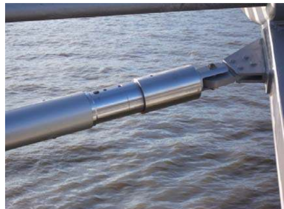
FIGURE 5 MOVING END OF PIER DAMPER
