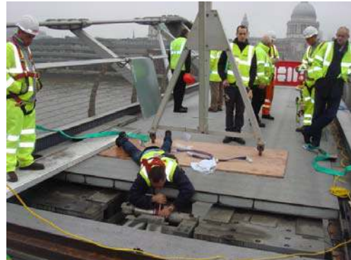
FIGURE 7 DECK DAMPER SHOWN WITH DECK PANELS REMOVED
