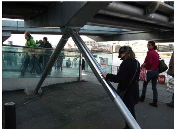
FIGURE 9 VERTICAL DAMPER PAIR WITH PEDESTRIAN ACCESS
