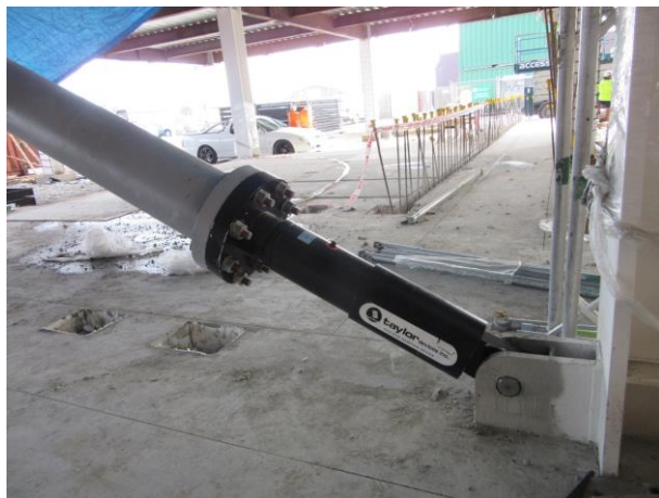
Figure 9: Frame with the viscous dampers in place
