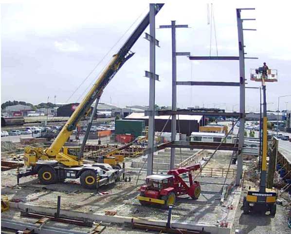
Figure 8: Erection of columns
