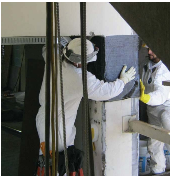
Figure 15 – Column confinement FRP installation.
