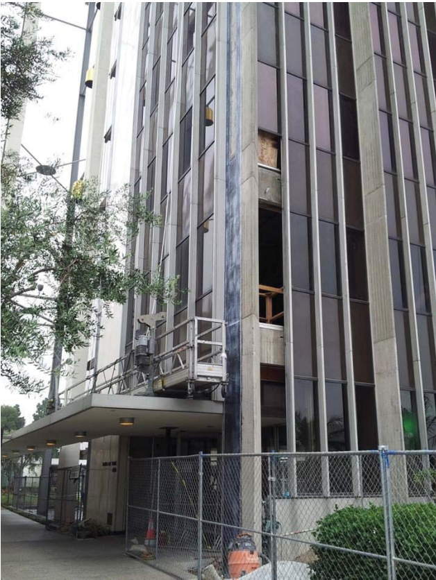
Figure 14 – Tower of Hope entrance with FRP visible on exterior face of concrete column.
