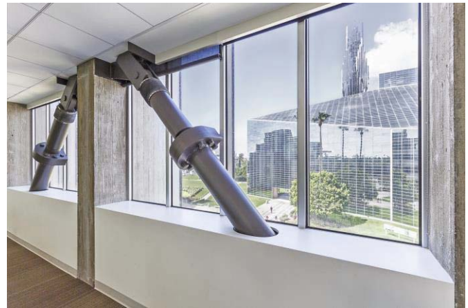
Figure 11 – Fluid viscous dampers on the north side of the Tower of Hope.
