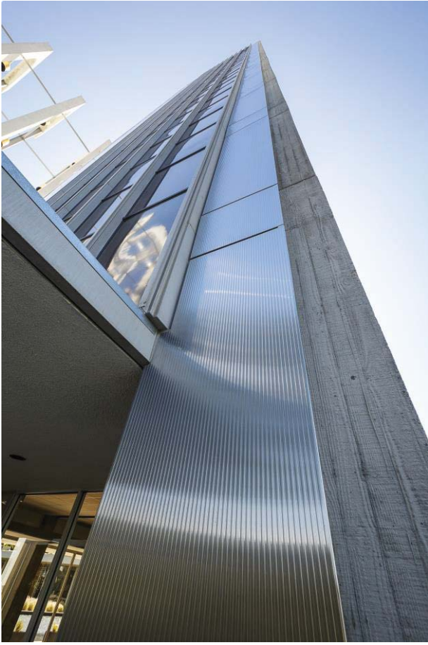
Figure 18 – Architectural metal paneling to hide FRP at column adjacent to building entrance. Reference Figure 14.
