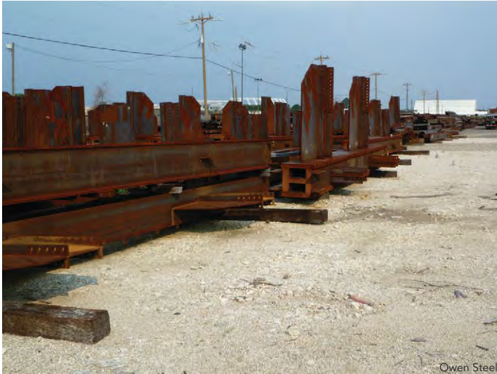
▲ Much of the project's steel resided at fabricator Owen Steel's storage yard while construction was on hold.
