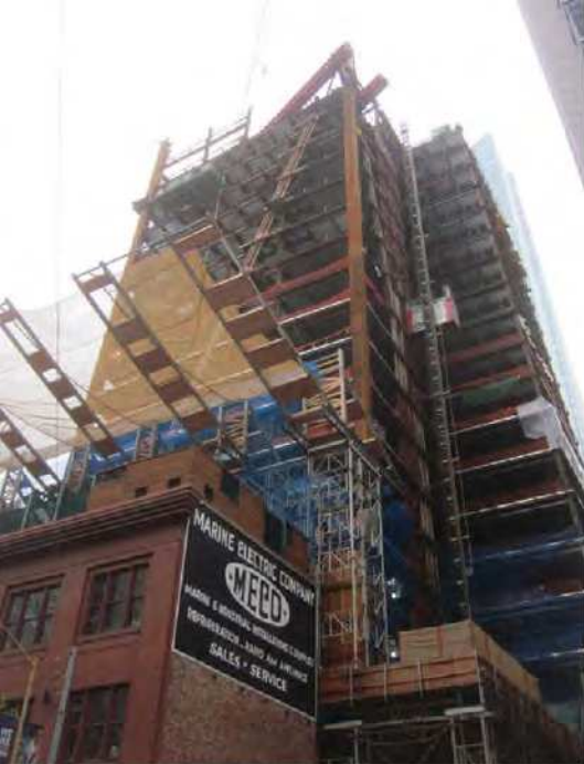
▲ A cantilevered safety net protects an adjacent building.
