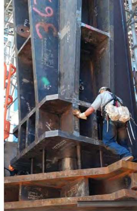
▲ Steel could only be erected from Fremont Street, and an assist crane was used for heavier picks at the back of the building.
