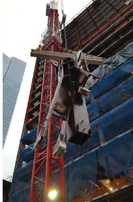
▲ Steel could only be erected from Fremont Street, and an assist crane was used for heavier picks at the back of the building.
