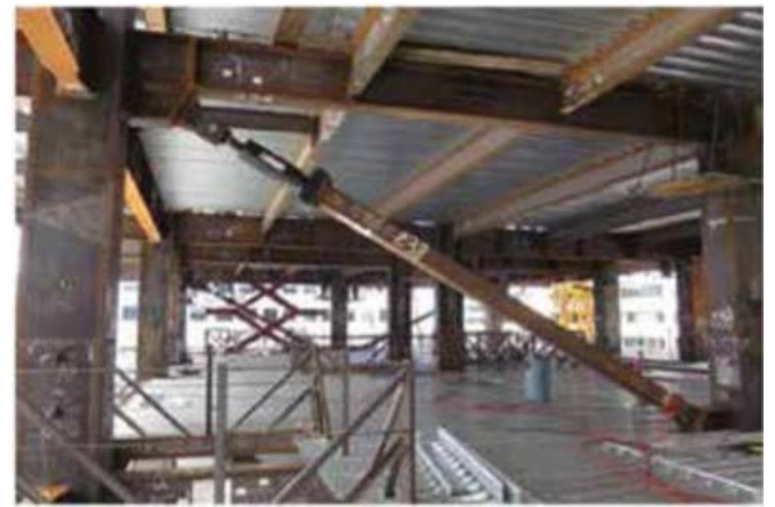
Typical installed VDD & Extended Braca
