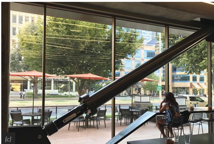
Figure 2 Example Buildings with FVDs (a) 12 Moorhouse Ave., Christchurch, NZ; (b) Damper with integral extender at 350 California, San Francisco, CA; (c) Damper in coffee house at 555 Capitol Mall, Sacramento, CA; (d) Criterion Promenade, Santa Monica, CA.
