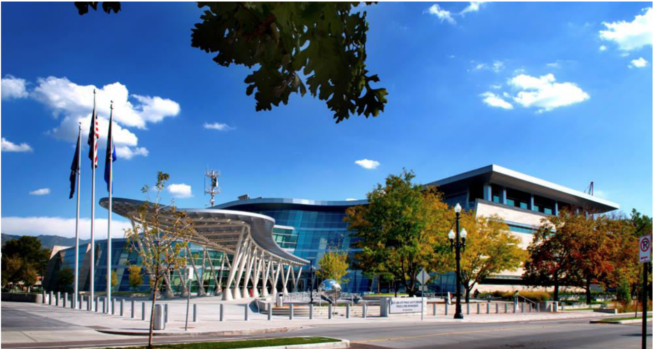
Figure 4. Salt Lake City Public Safety House building
