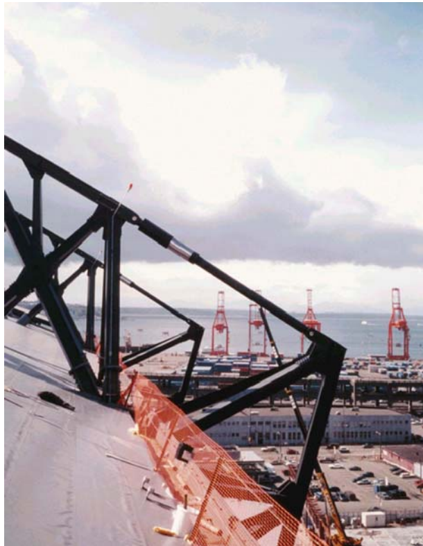
FIGURE 37 DAMPER INSTALLATION AT THE PACIFIC NORTHWEST BASEBALL STADIUM
