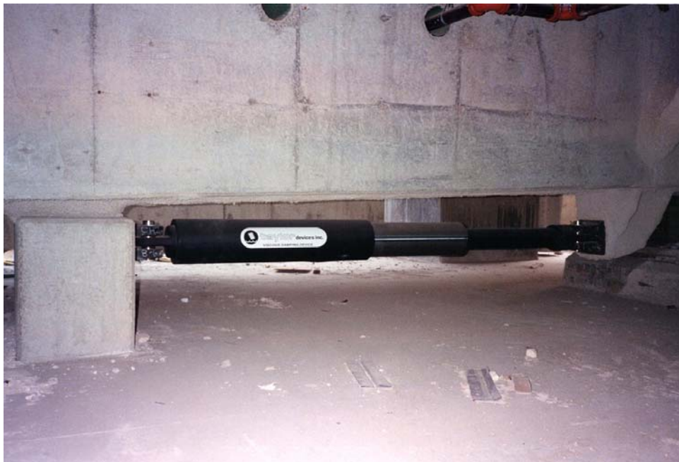
FIGURE 27 ARROWHEAD REGIONAL MEDICAL CENTER INSTALLATION OF DAMPER
