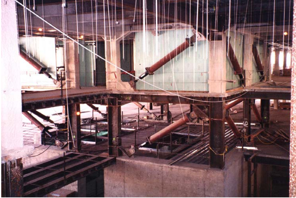
FIGURE 30 SAN FRANCISCO CIVIC CENTER DAMPER INSTALLATION
