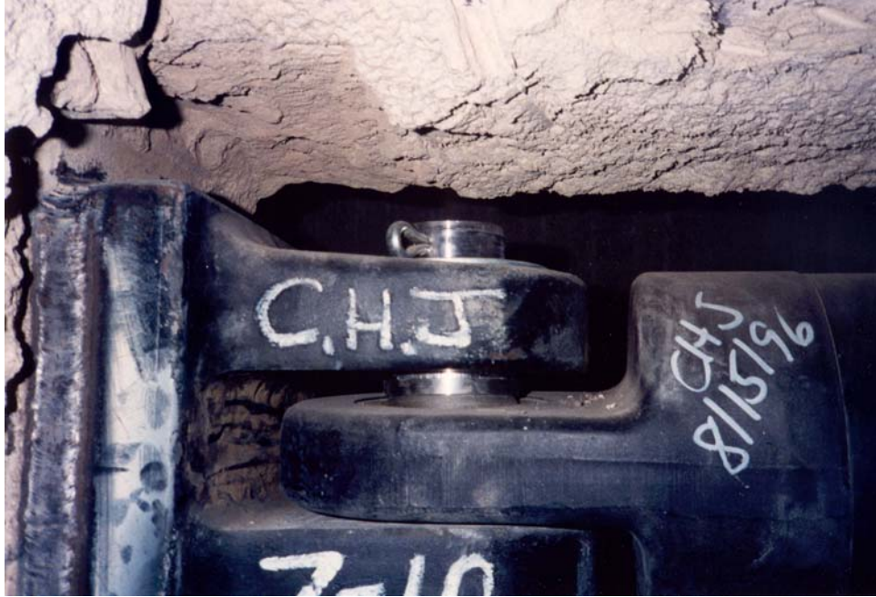
FIGURE 28 ARROWHEAD REGIONAL MEDICAL CENTER CLOSEUP OF ATTACHMENT OF DAMPER
