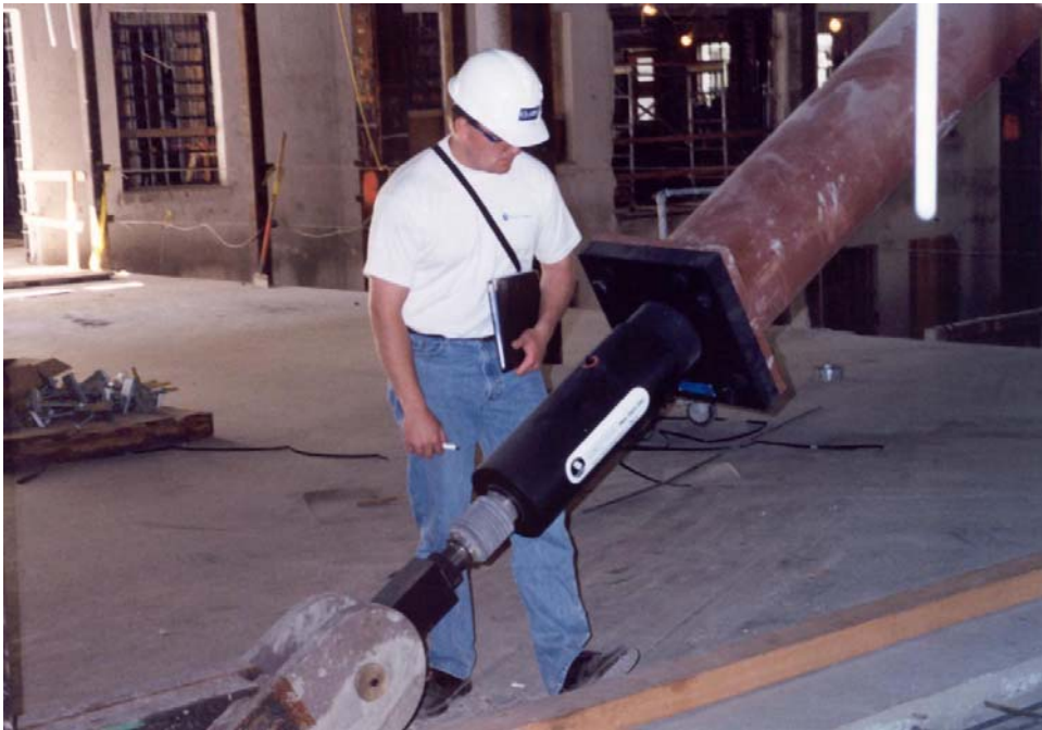
FIGURE 31 SAN FRANCISCO CIVIC CENTER DAMPER CLOSEUP SHOWING CONNECTION DETAILS
