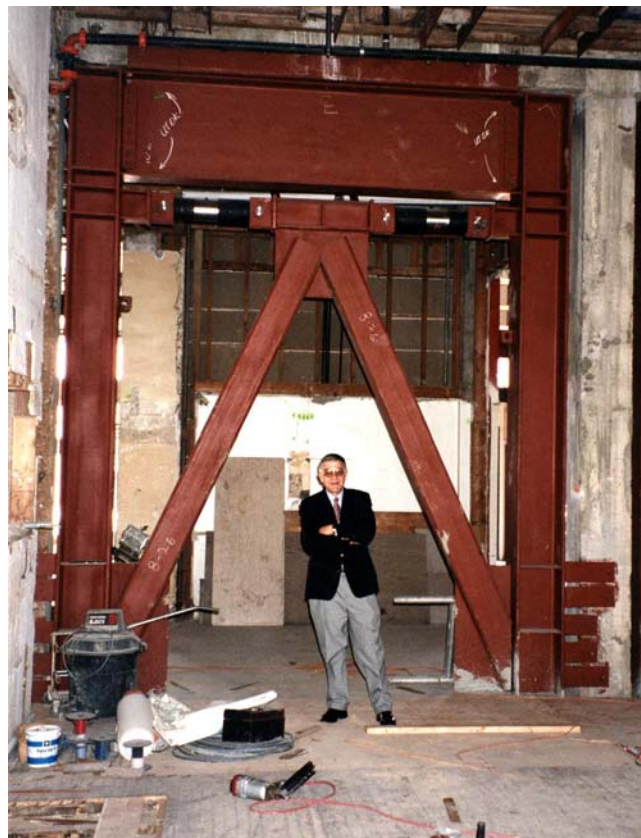
FIGURE 33 HOTEL WOODLAND - INSTALLATION OF DAMPERS
