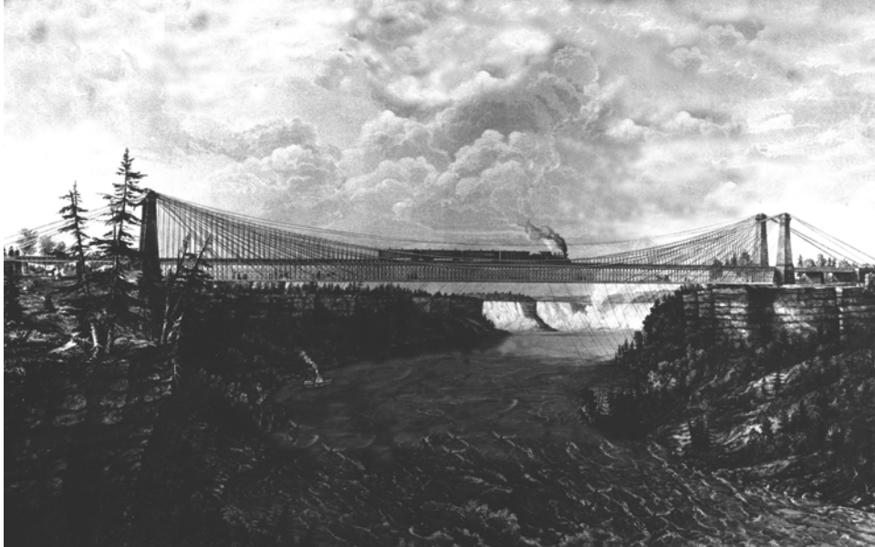
FIGURE 2 JOHN ROEBLING'S RAILWAY SUSPENSION BRIDGE AT NIAGARA FALLS, NY - 1854
