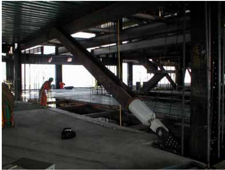
FIGURE 13 DAMPER INSTALLATION
