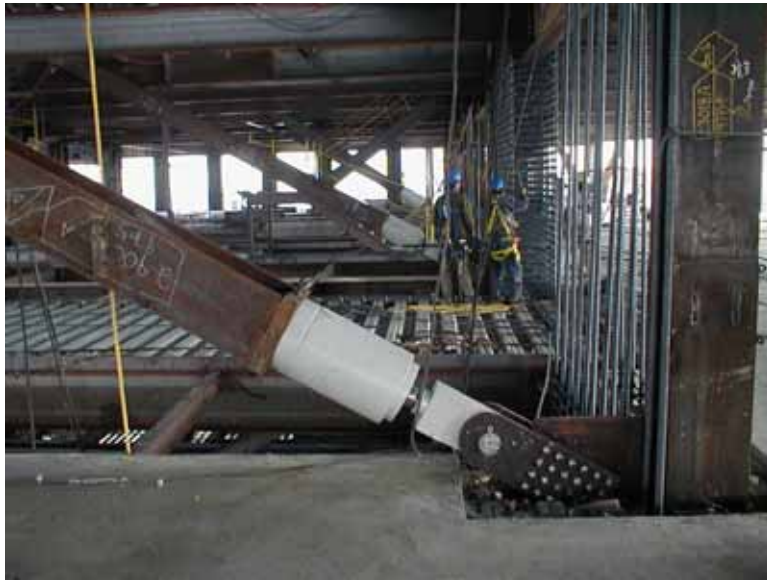
FIGURE 12 DAMPER INSTALLATION
