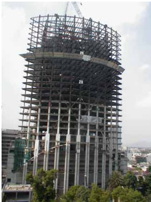
FIGURE 8 TORRE MAYOR BUILDING FRAME
