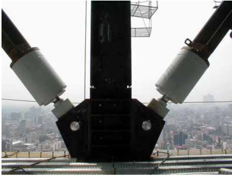
FIGURE 11 DAMPER INSTALLATION
