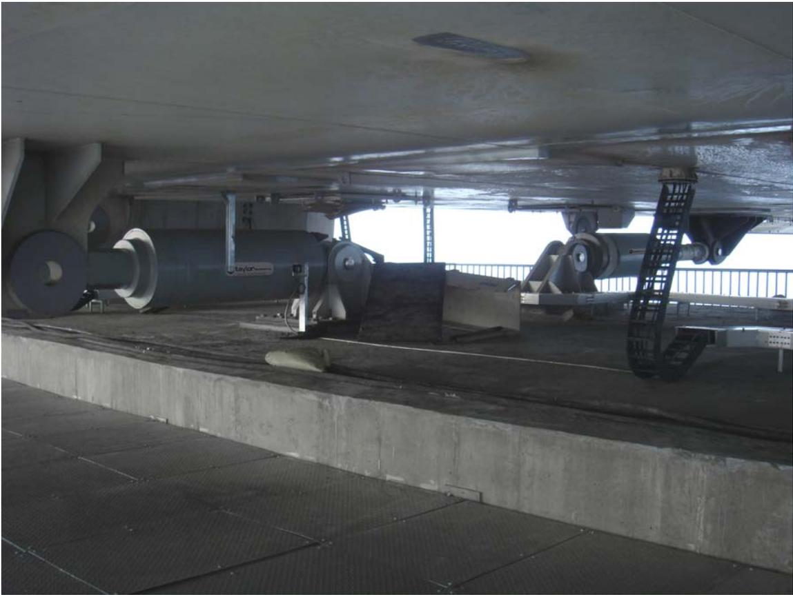
**Figure 21 – Isolators Installed on Sutong Bridge**
