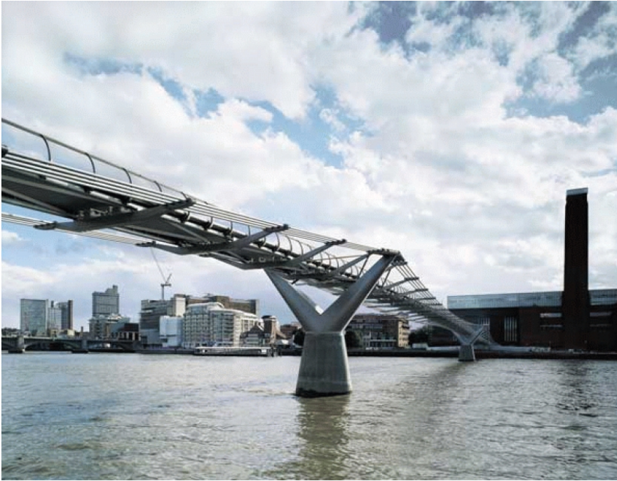
Figure 4 : The Millennium Bridge
