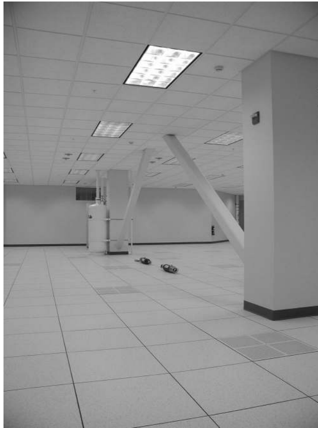
Figure 11. Typical interior clean room.
