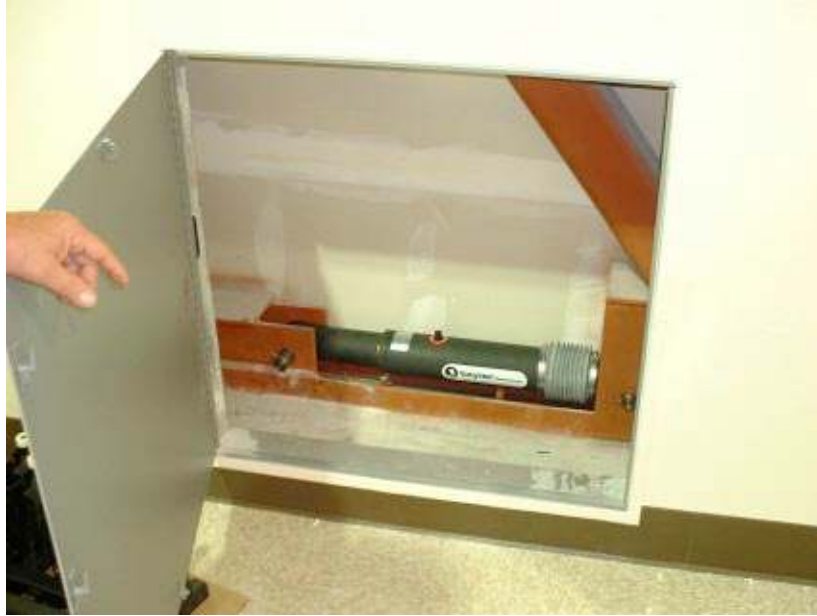
Figure 9. Typical damper installation.
