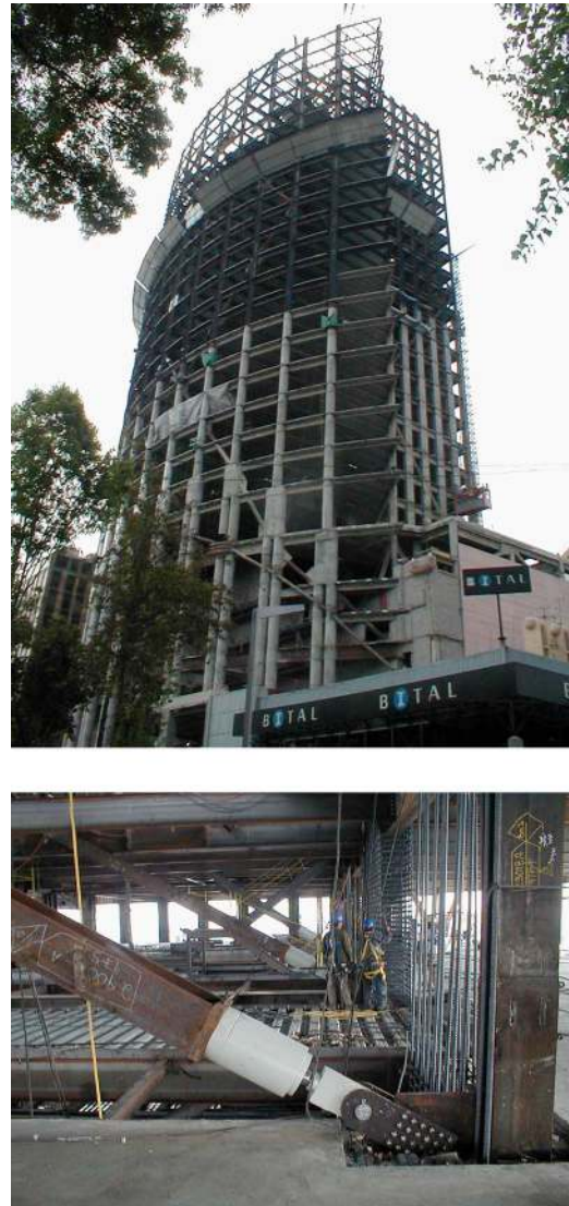
Fig. 6. Photos of: (a) Torre Mayor Tower under construction showing partial view of megabraces; (b) closeup view of installed fluid dampers (Photos courtesy of Taylor Devices, Inc.)
