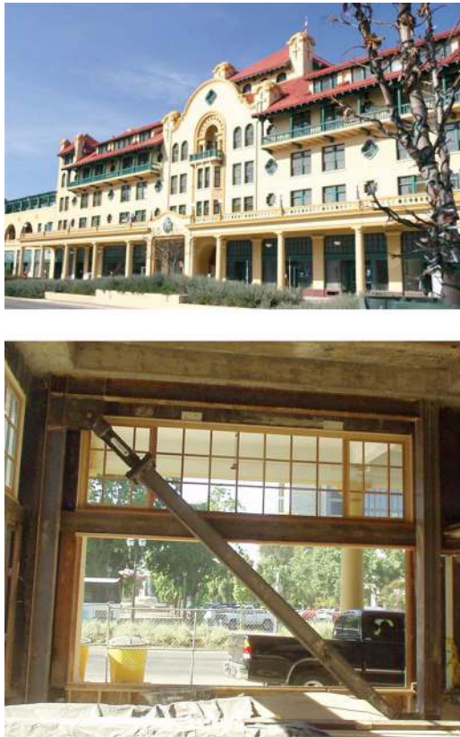
Fig. 5. Photos of: (a) renovated Hotel Stockton; (b) view of installed fluid viscoelastic damper (Photos courtesy of Miyamoto International, Inc.)
