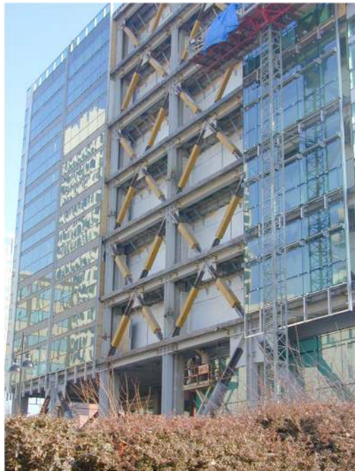
Fig. 7. Photos of: (a) Wallace F. Bennett Federal Building; (b) view of building without cladding showing installed buckling-restrained braces (Photos courtesy of SIE Corp.)
