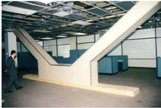
Fig. 11. Photos of: (a) LAPD Recruit Training Center; (b) view of chevron brace assembly containing viscoelastic damper at floor level (Photos courtesy of The Crosby Group and SIE Corp., respectively)
