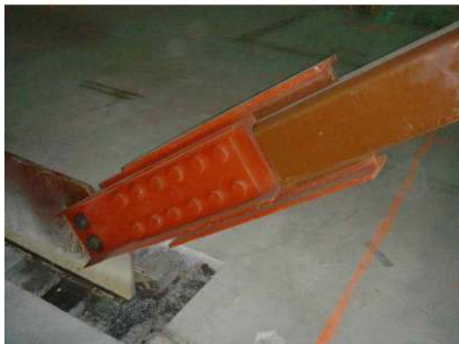
Fig. 9. Photos of (a) Monterey County Government Center showing precast concrete panel cladding; (b) closeup view of installed friction damper [Reprinted from Chang et al. (2006), with permission from Earthquake Engineering Research Institute]
