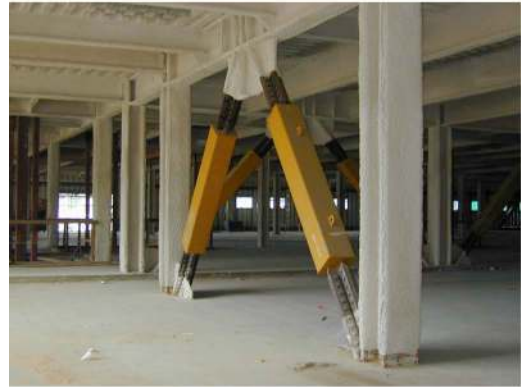
Fig. 8. Photos of: (a) Santa Clara Medical Center Hospital under construction; (b) closeup view of installed buckling-restrained braces (Photos courtesy of SIE Corp.)
