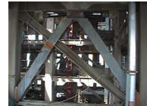
Fig.8 Cross Brace Damper
