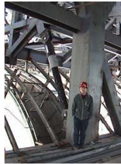
Fig.7 Installed 1500kN Damper
