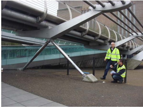
FIGURE 8 INSPECTION OF VERTICAL DAMPER PAIR
