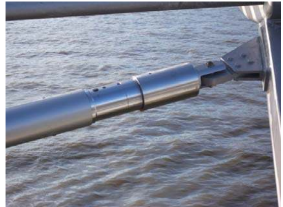
FIGURE 5 MOVING END OF PIER DAMPER OVER THE RIVER THAMES
