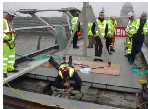
FIGURE 7 DECK PANELS REMOVED DECK DAMPER SHOWING
