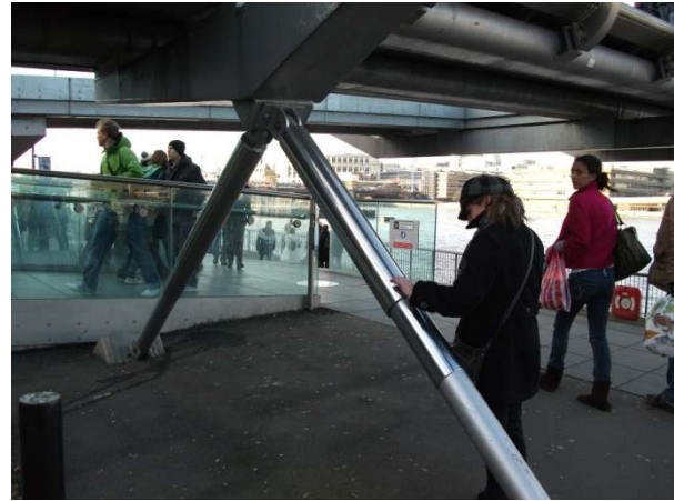
FIGURE 9 VERTICAL DAMPER PAIR WITH PEDESTRIAN ACCESS
