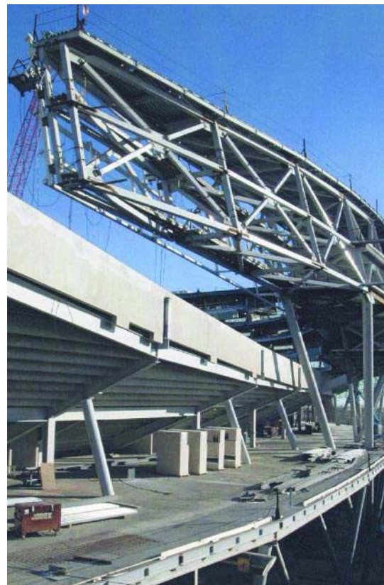
To accelerate the steel fabrication and erection process, designers used Xsteel 3D-modeling software. Xsteel produces a full-size, annotated computerized model. Once the model is created, piece drawings for fabrication and general-arrangement drawings can be produced automatically.
