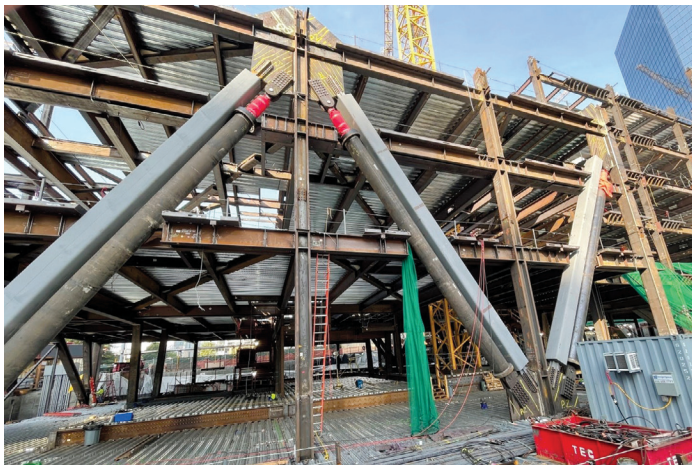
The super brace buckling restrained brace and damper system on The Artise (photo by Scott Erickson).
