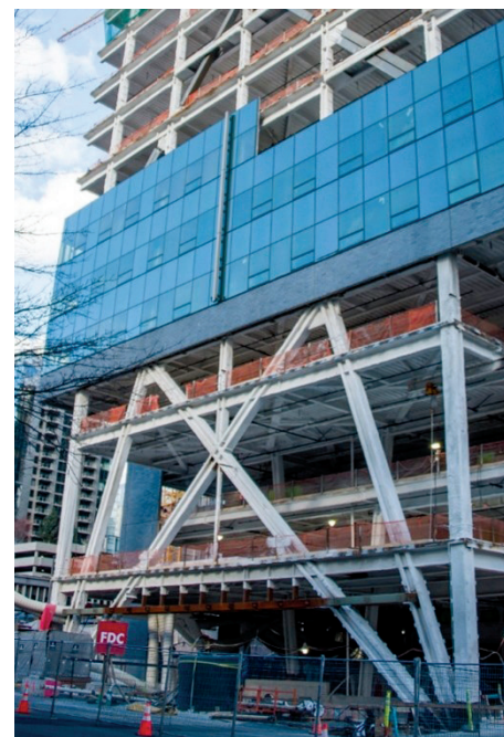
West lateral frame during construction (Photo by Scott Erickson)
