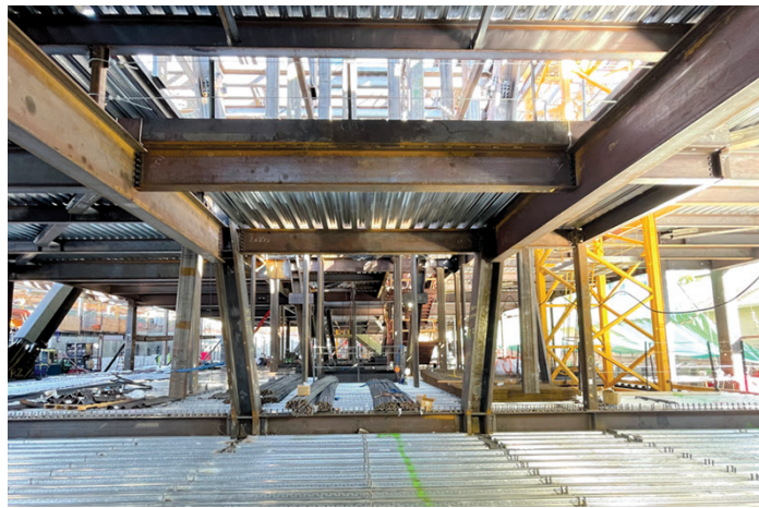
Internal sloping columns during construction (photo by Scott Erickson)
