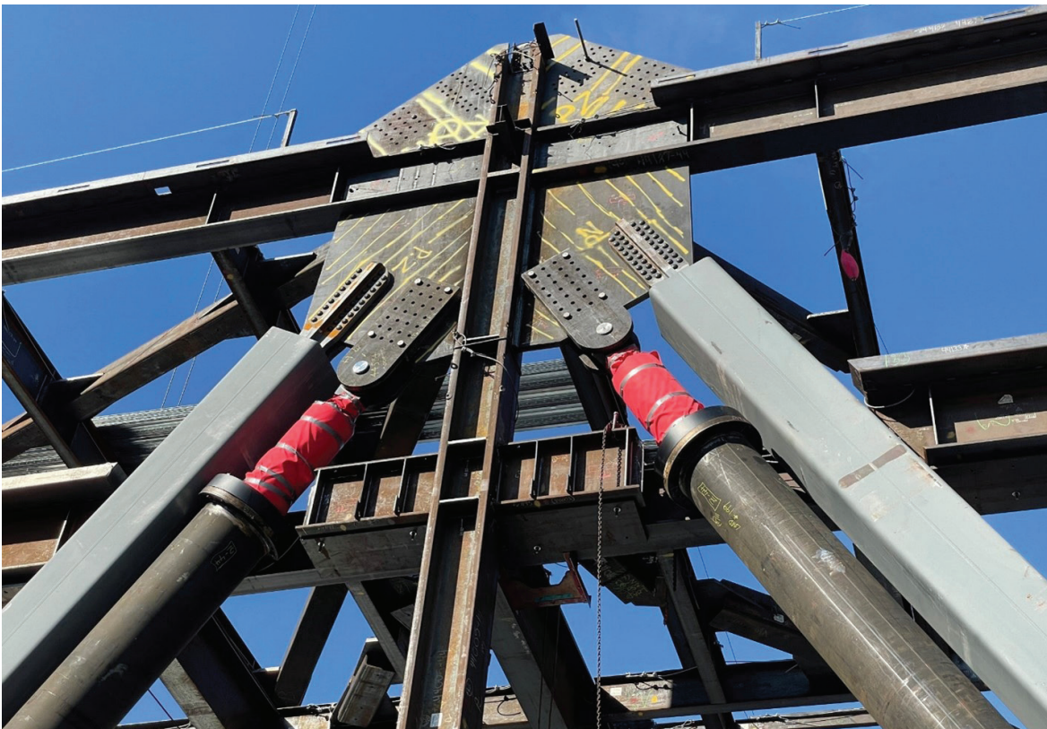
Damper and buckling restrained brace system on The Artise (photo by Scott Erickson).
