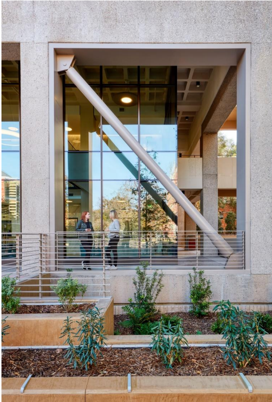
Figure 9. Installed Damper in Concrete Frame (UCLA Franz Hall)
