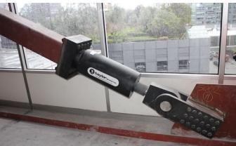
Sometimes shim plates (as seen below) are used to provide further length adjustment. Single shim plates or multiple shim plates can be used. Shim plates up to 1 inch (25mm) thick have been used between the damper and the (contractor supplied) HSS extender brace.
