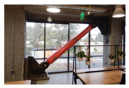
The telescoping damper is welded around the perimiter of the nested "telescoping" tubes after installation. The multi piece design allows this style of damper to be brought into the building in pieces that can be designed to fit into a service elevator.
